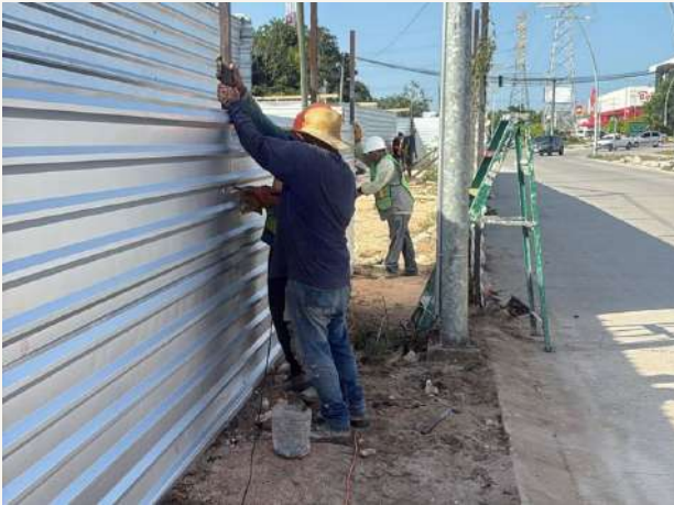
01 • Preliminary works and site enclosure
