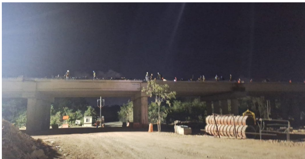
Night work on the elevated viaduct.
