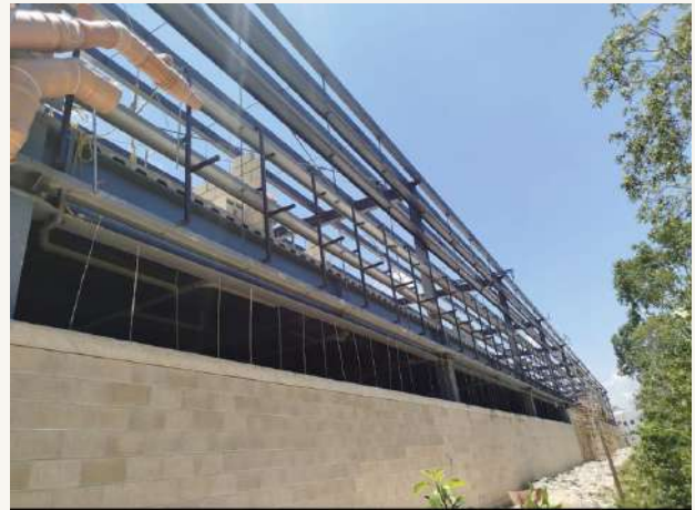
04 • Structural steel and roof erection
